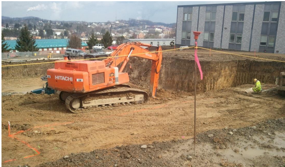
Figure 1: Site Excavation (Courtesy of Owner)
